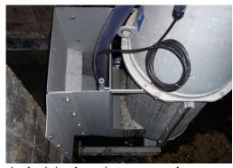
Oostburg's RoK4 has required minimal repair or parts replacement with only one set of auger brushes replaced over its six year lifetime.
